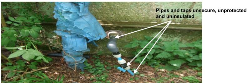
Outlet pipes at the bottom of the tank: Right; pipe supplying the most northerly property of Claverhambury via isolated supply pipe; Left; pipe supplying all other properties
